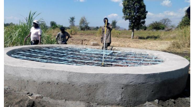
A completed seepage well in Malawi
